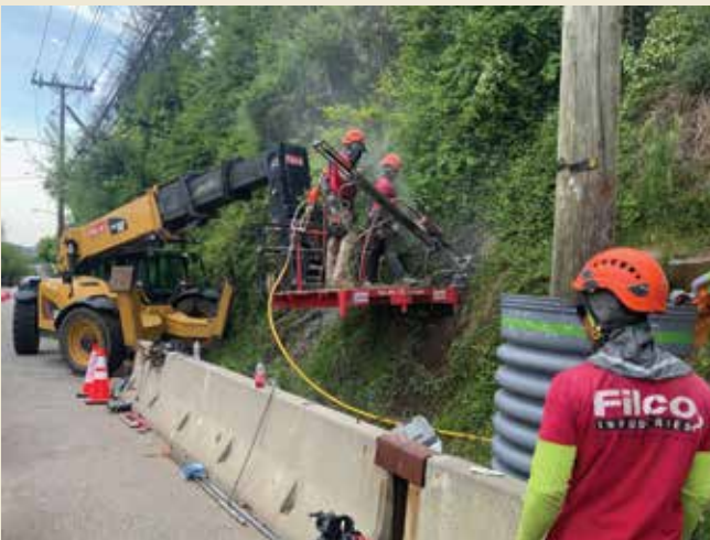
Filco’s custom equipment allows crews to work where conventional methods can’t.
