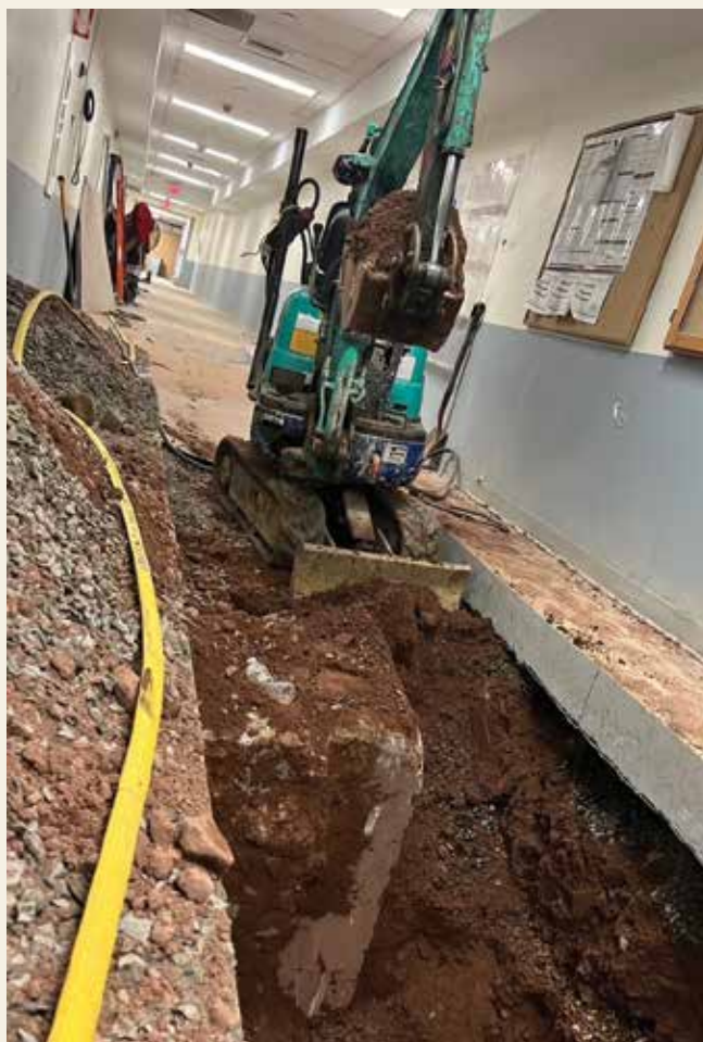
Compact equipment allows Filco crews to work inside occupied buildings.
