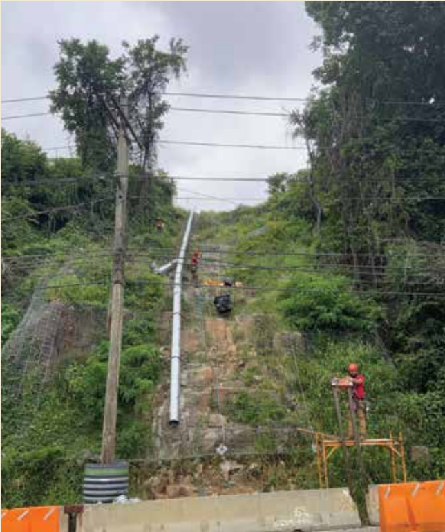
Specialized equipment helps crews safely complete projects on steep terrain.
