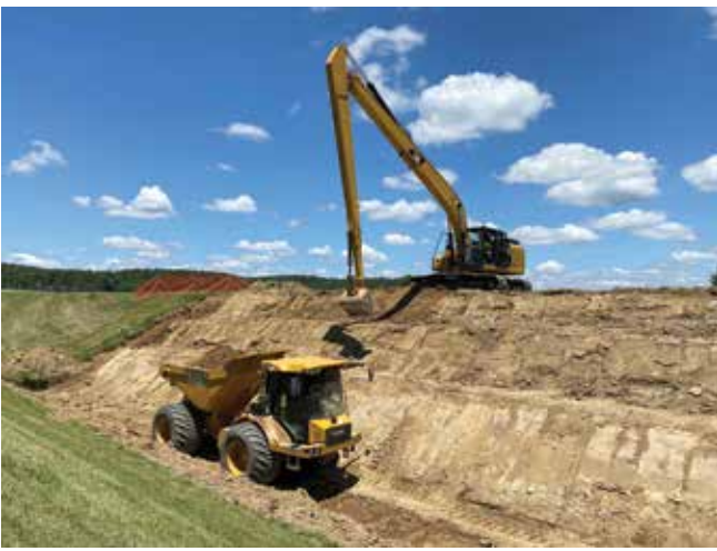
Brannon Contracting long-reach excavator in action.
