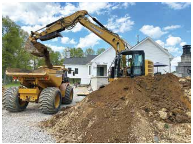
Dustin's son Beau operating one of the company's excavators.
