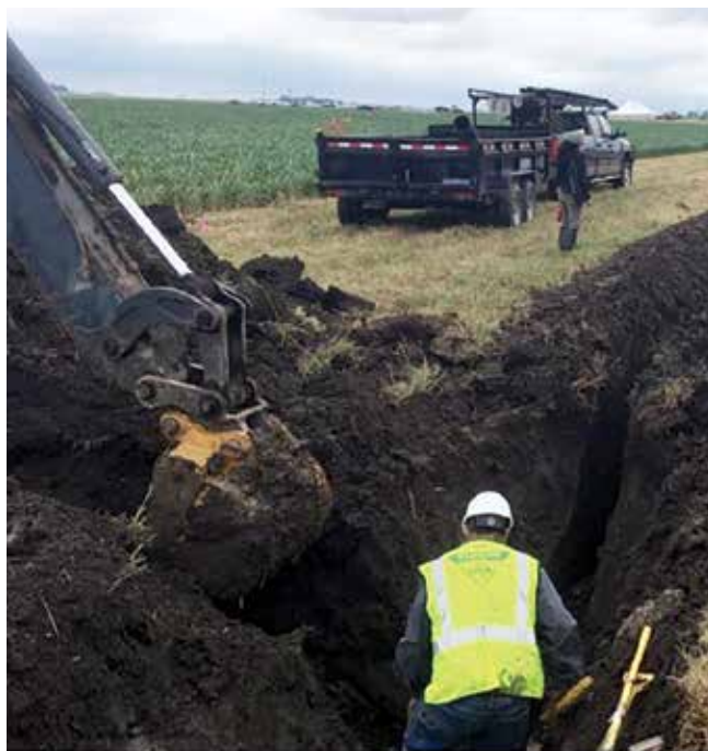
Illinois LICA installing a saturated buffer at an Illinois Sustainable Ag Partnership and ADMC partnered field day.
