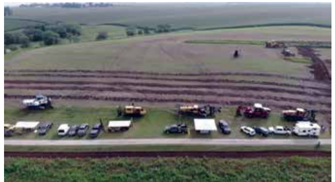
Tiling project on the Iowa LICA Farm
