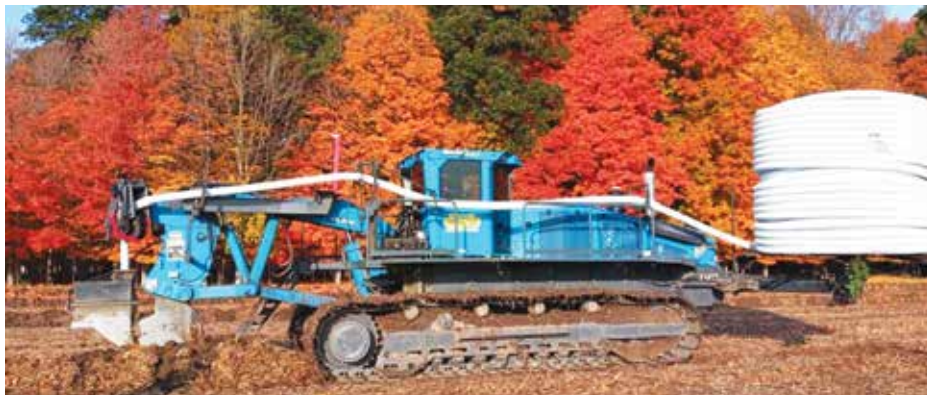
Tile installation on a beautiful fall day.
