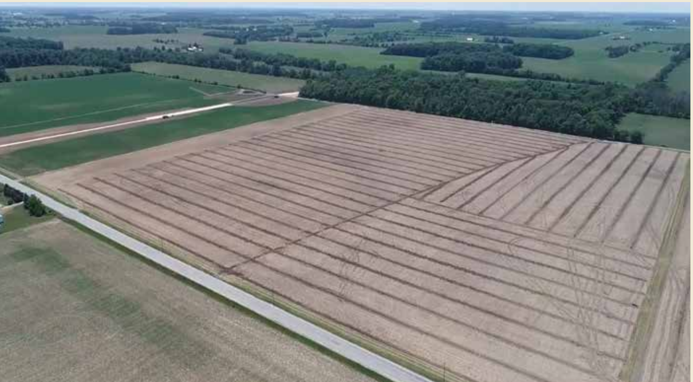
Completed tile work on the DPAC farm.
