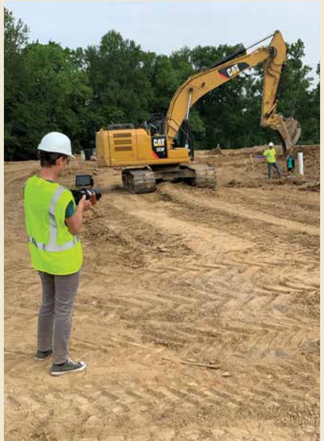
Filming the job site for the video.
