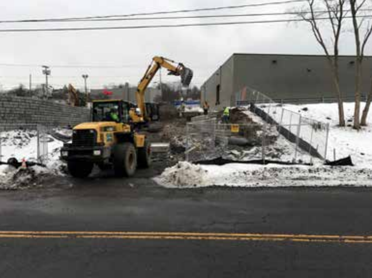
Retaining Wall, Tipp Hill, NY
