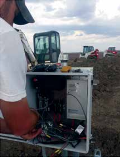
Waterborne Environmental technician, Scott Cleary, installs instrumentation at the field laboratory. Image courtesy of Waterborne Environmental
