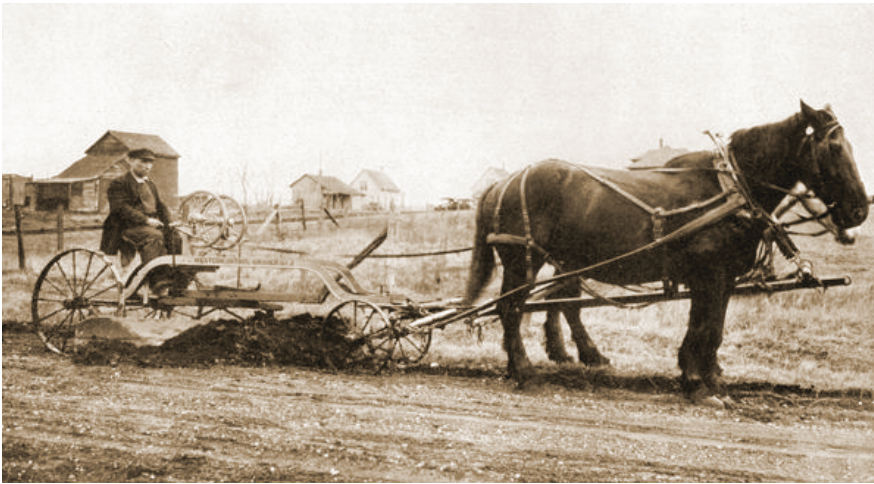
Western Patrol Grader No. 2, from 1925 Austin-Western Road Machinery Company catalog, HCEA Archives.
